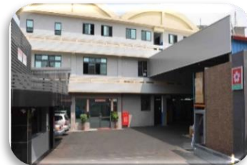
Shenkang plant Rang Hood
