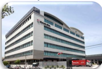
Daya plant I Dish Dryer
